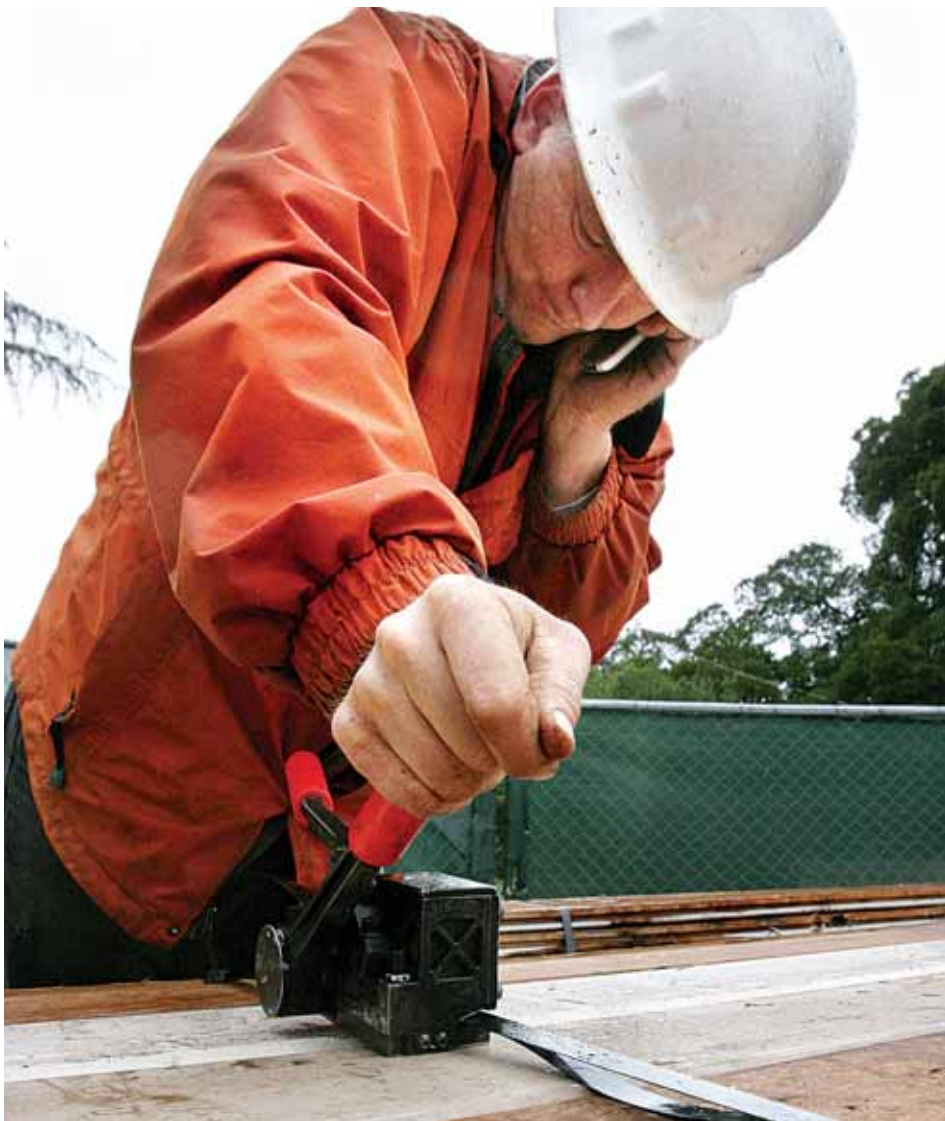
Jim Steinmetz of Reusable Lumber Company bands units of lumber using a banding machine at the former site of Portola Valley Town Center.
