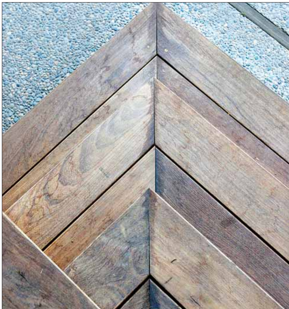
A close-up of ipe, an ironwood grown in Central and South America.
