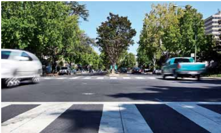
California Street at its intersection with Franklin Street.
