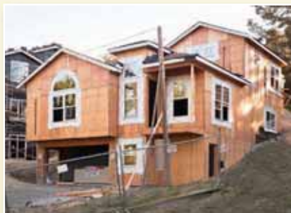
Construction site as of 10/27/11
