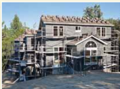
Construction site as of 10/27/11 Rear elevation shown
