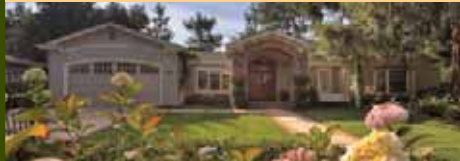
PINECREST DR, LOS ALTOS Custom remodel/expansion. $2,725,000.
