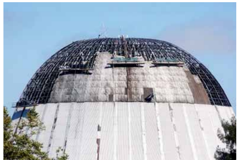
At left: Dismantling of the hangar's siding started April 18, 2011. At right: Beneath the toxin-laced siding, a layer of redwood is revealed.
