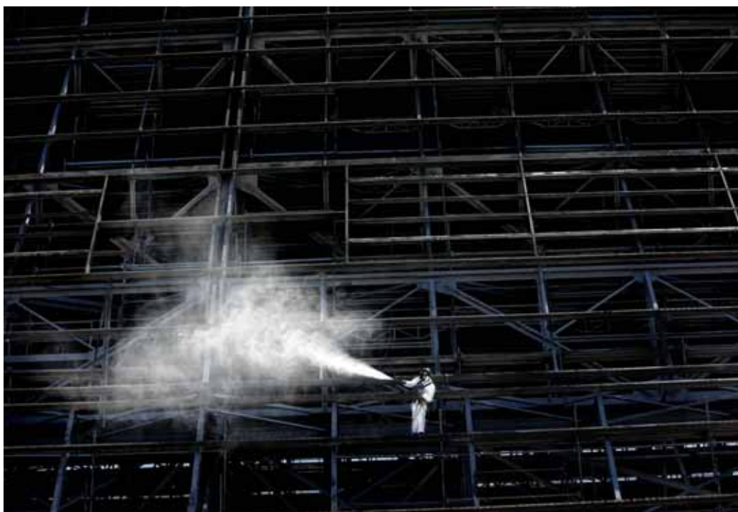
Clockwise from top: Two workers with a bird's-eye view of the stripped hangar; workers remove the last pieces from hangar's roof on July 19; wearing protective gear, a worker uses a high-pressure hose to clean the skeleton.
