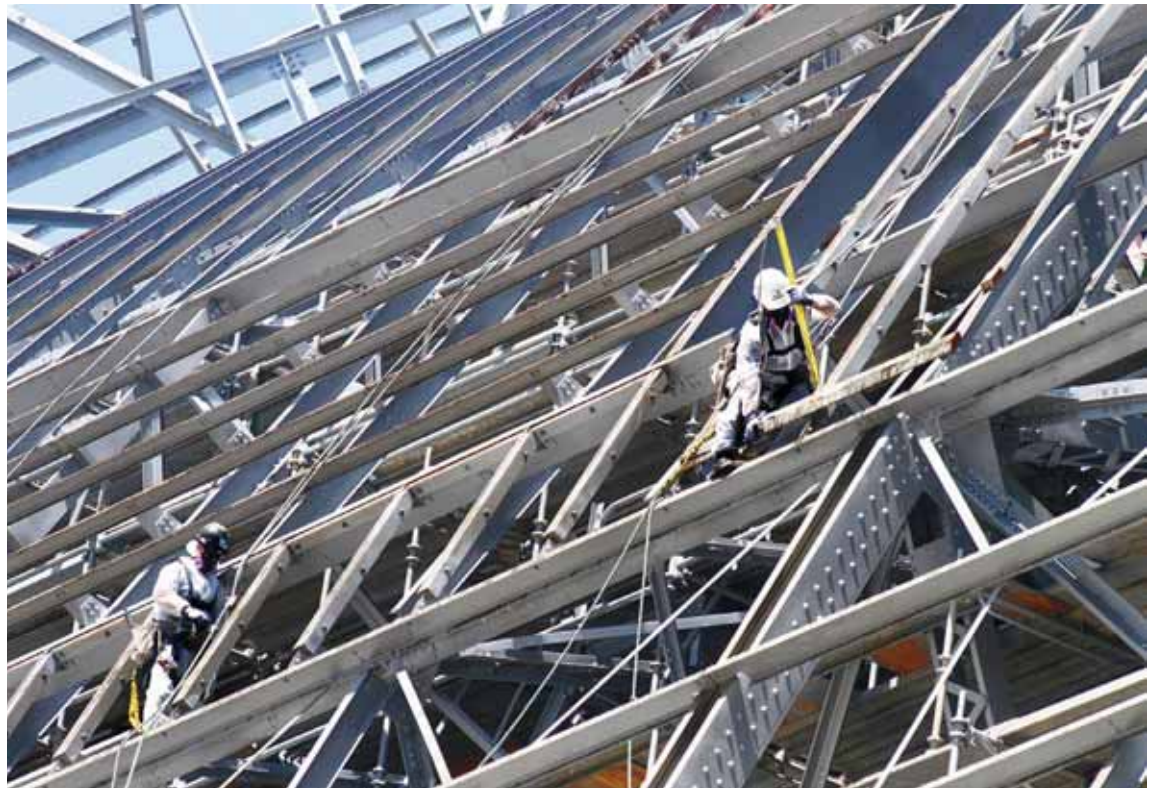
Workers remove the last piece of Hangar One's siding in late July.
