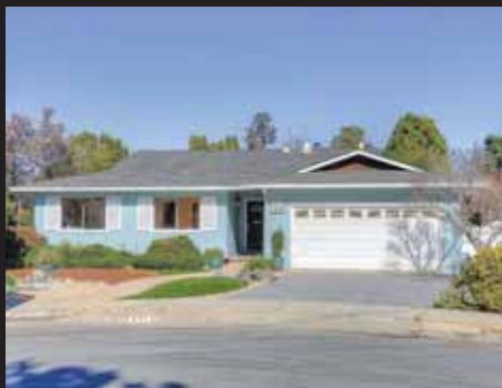
331 JARVIS COURT, SUNNYVALE
